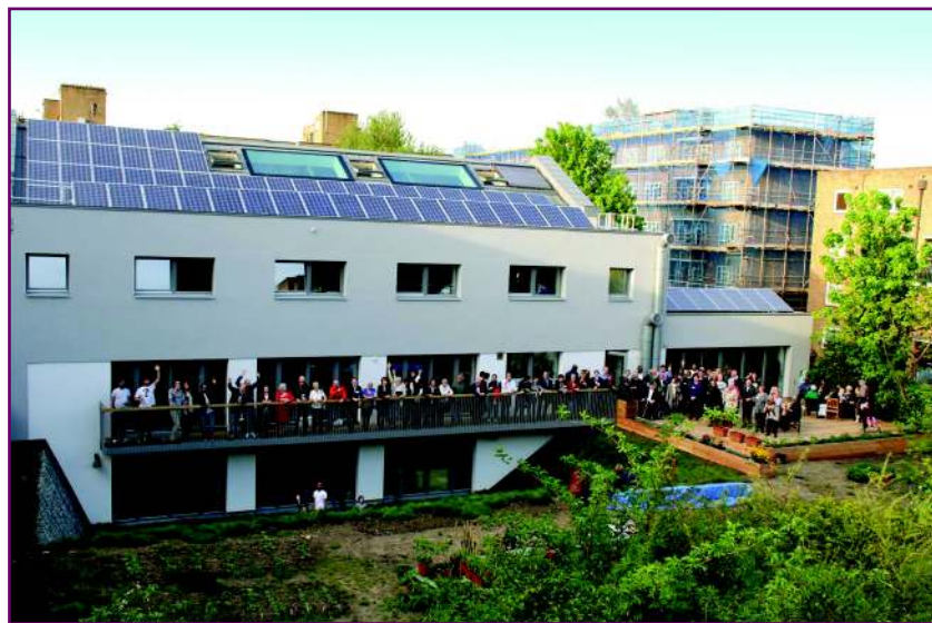
The Mildmay Community Centre has demonstrated that the very low energy standards of Passivhaus can be achieved in the UK. But this only not only requires attention to detail in design but also very good project management on site to ensure that all the details are constructed correctly.
