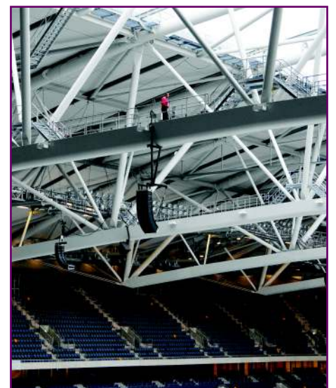
Figure 1: Primary roof trusses of the Friends Arena Stockholm.
